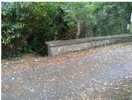
Plate 14.14 Bridge over townland boundary,
