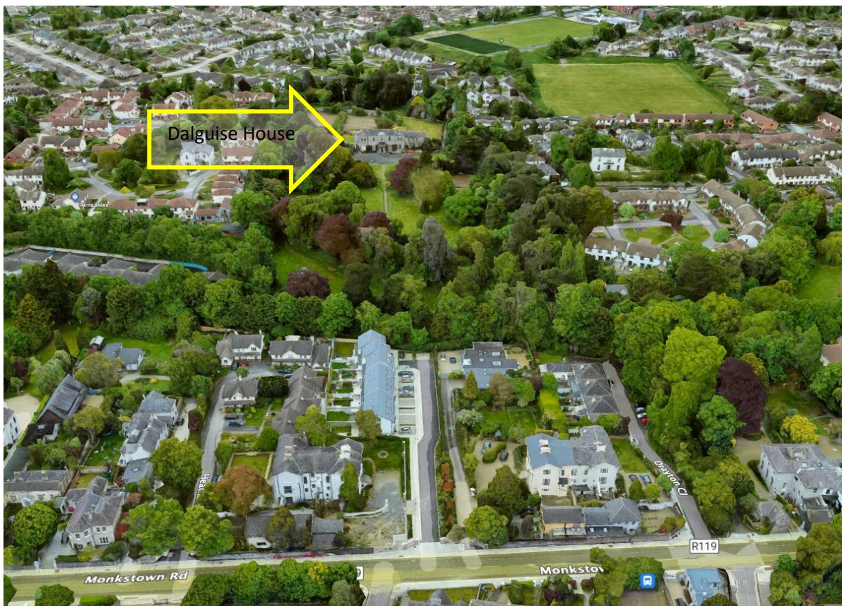
Figure 13.1 – Dalguise site looking south from above the coastline.
