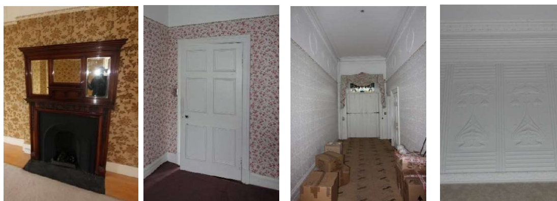
Fig.15.16: Late 19 th century fire piece (L), typical door joinery (M), cornice & frieze details (R)
