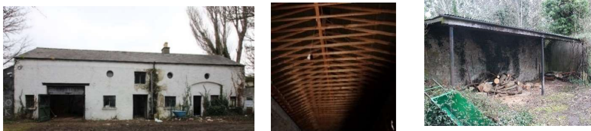
Fig.15.19: East elevation of stables (L), modern timber roof structure (M), Lean-to structure (R)
