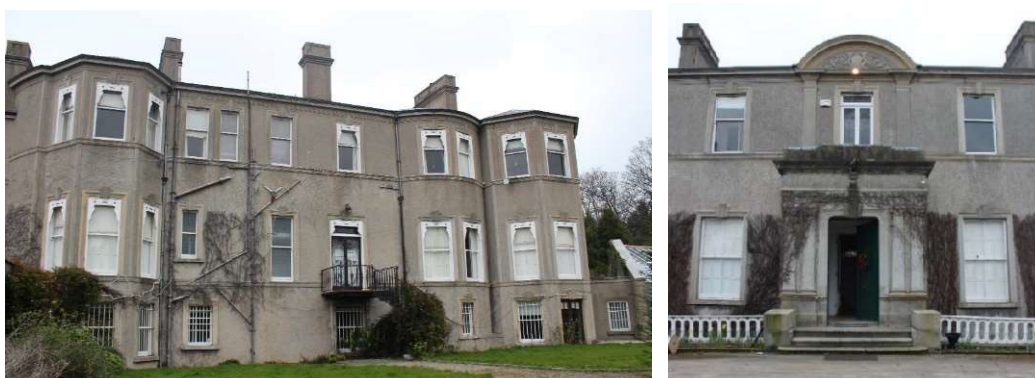
Fig.15.10: Rear Elevation (L), Entrance portico (R)
