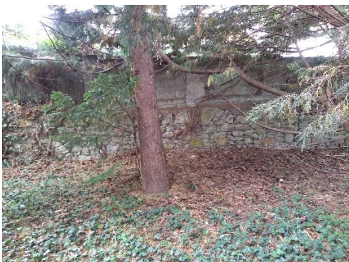
Plate 14.1 Southern wall, facing south
