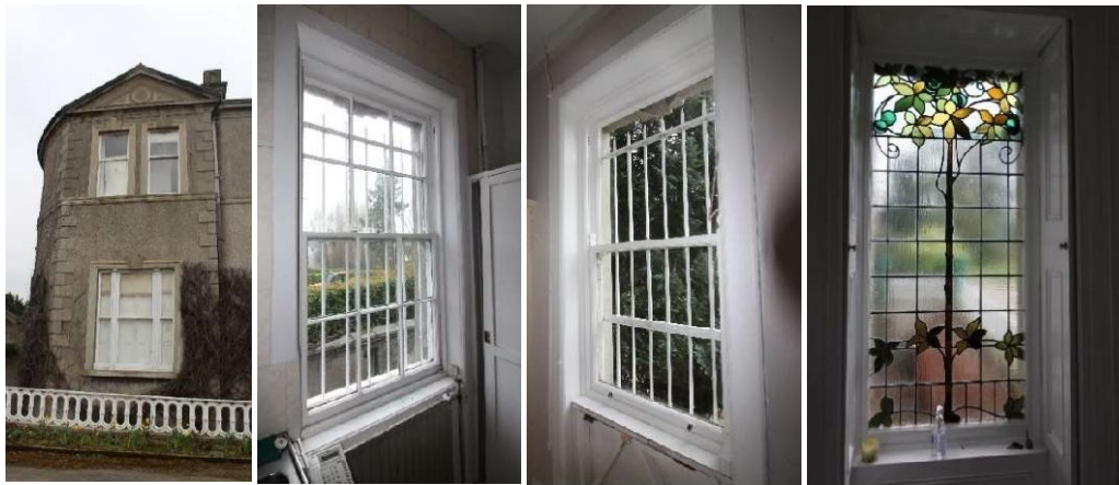
Fig.15.11: View of Wing (L), typical windows
