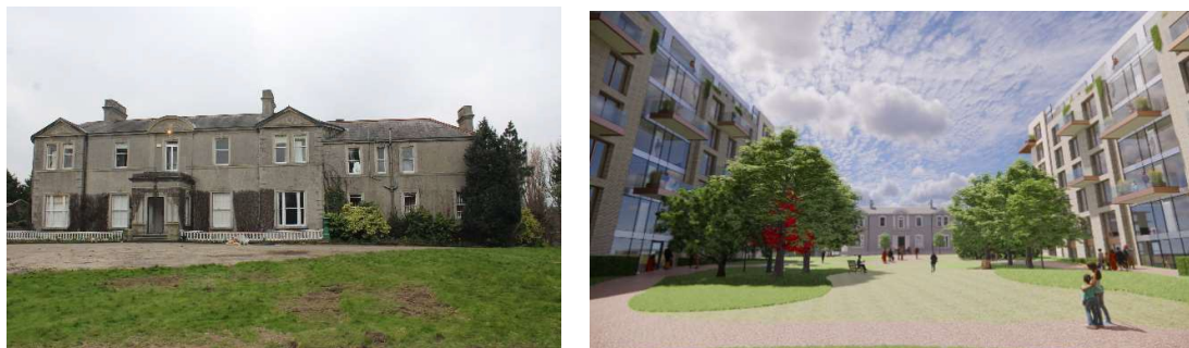
Fig.15.26: View toward front façade of Dalguse House
