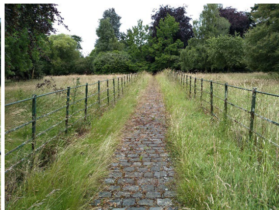
Plate 14.10 Pathway and railings, facing north
