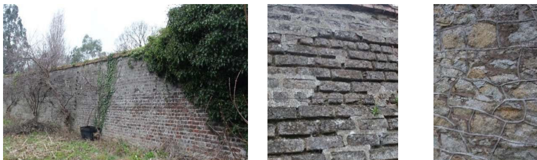
Fig.15.18: View of inner wall (L), detail of brickwork (M), rubble stone on outer surface (R)
