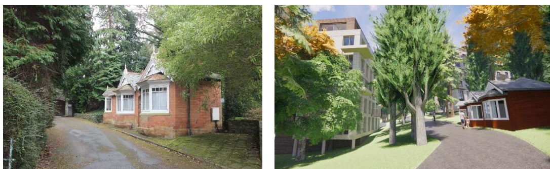
Fig.15.25: View looking east with Gate Lodge/Brick Lodge
