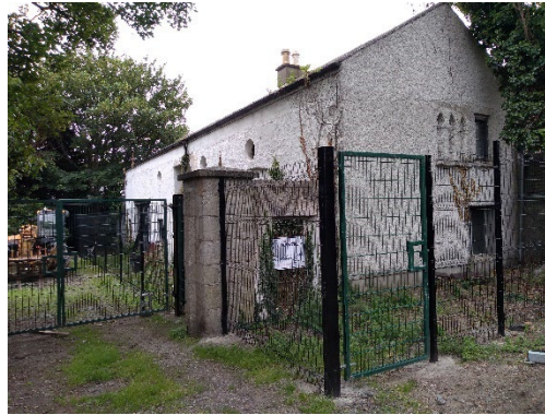
Plate 14.3 Coach house, facing southwest
